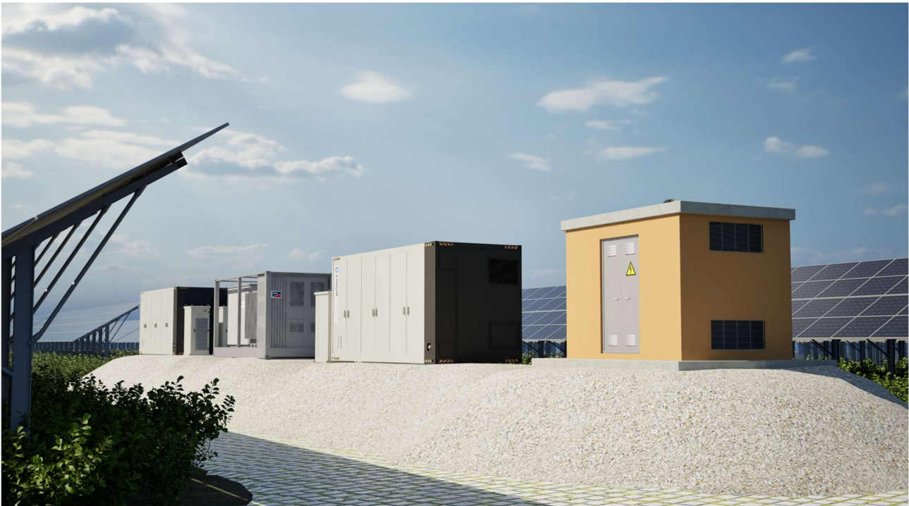
Figura 4-4: Rendering Cabinati Power Station, Container batterie e Cabina ausiliaria
