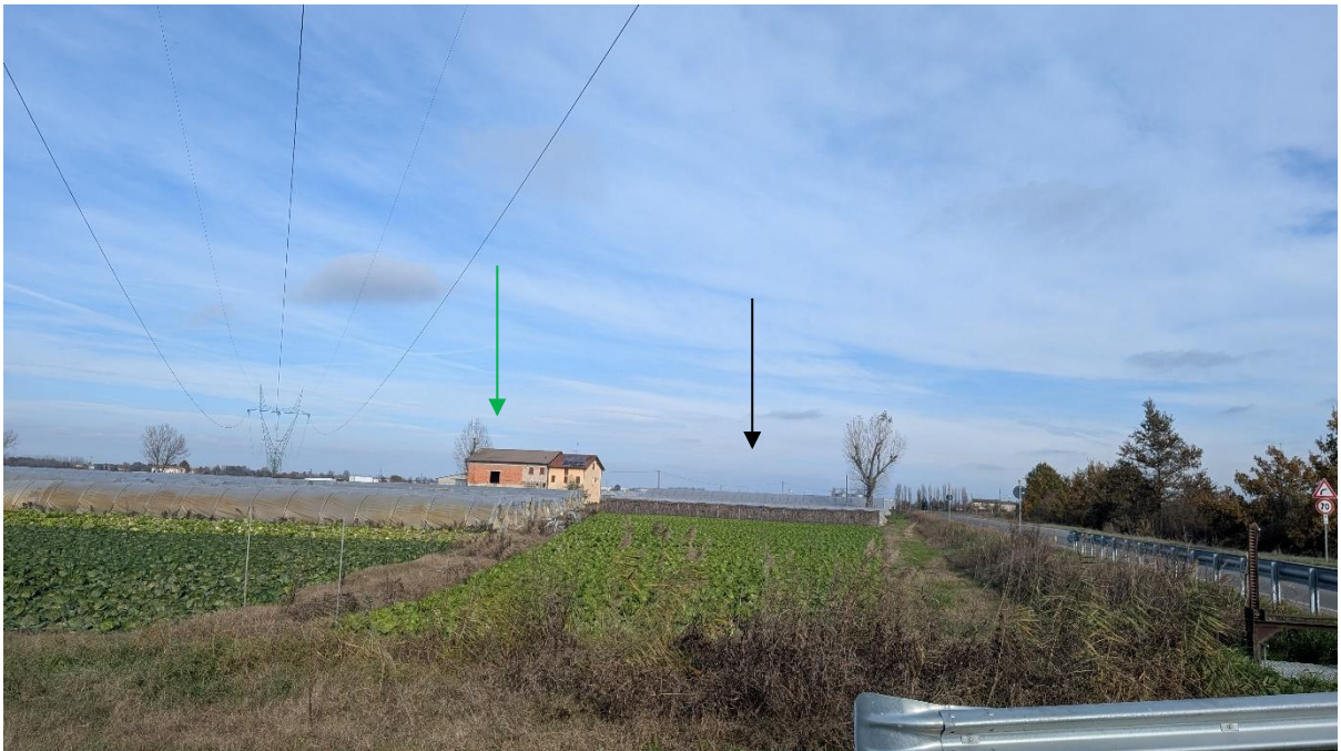
PdV 2 - SP 46 – post operam
